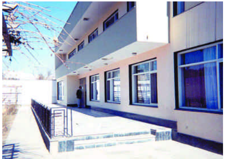
Emergency Loya Jirga Commission Headquarters
